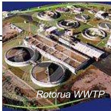
(2) Advanced WWTP land treatment
