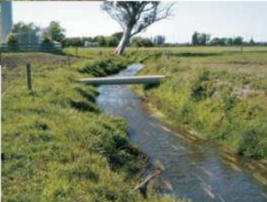
Fig 1b - Same drain as in fig 1a in autumn after weed removal
