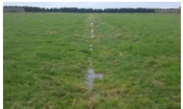
Shallow depression or swale channelling runoff into drain
