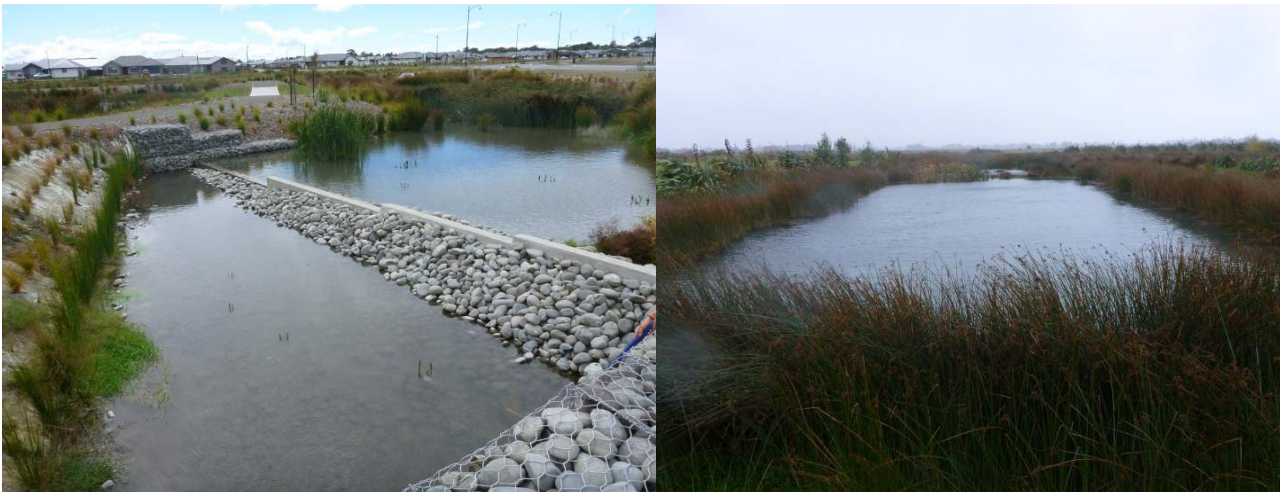
Figure 8: Constructed wetlands near Lincoln township.
