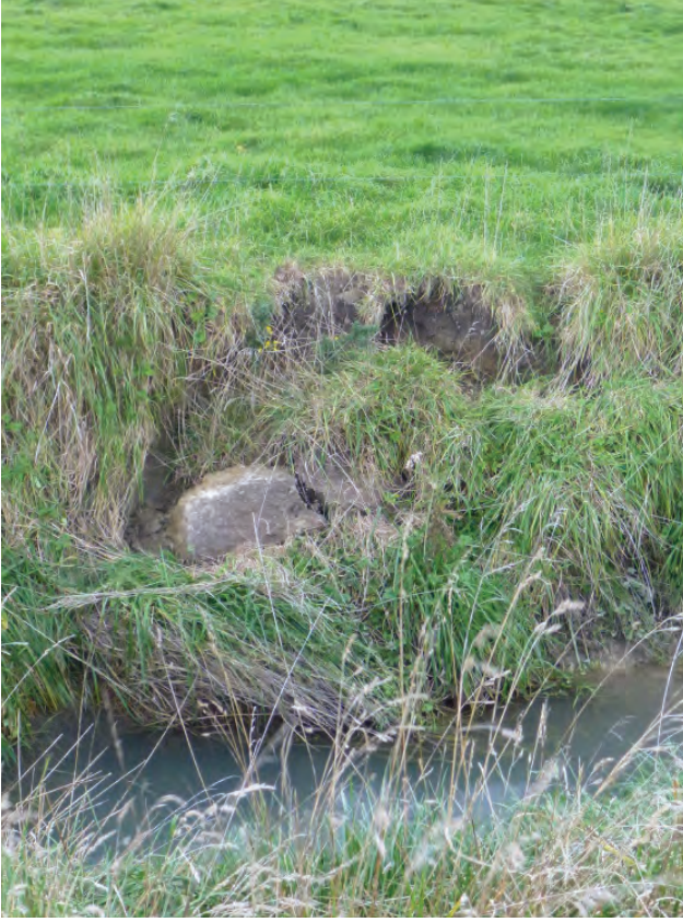
Stream bank slumping observed during the surveys
