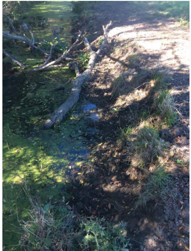
Complete lack of fencing and obvious stock damage
