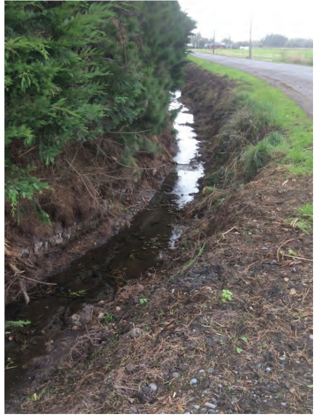
Drain condition immediately following drain maintenance
