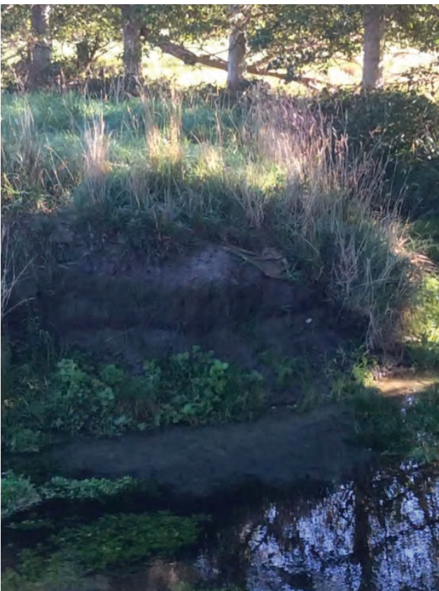
Bank slumping and erosion on the mainstem
