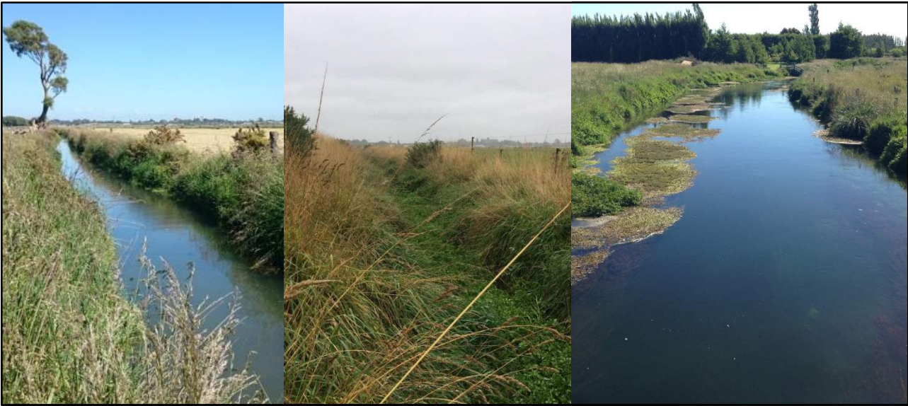
Figure 4: Typical Ararira / LII River waterways: Springs Creek (left); Lincoln Main Drain (centre) and Ararira / LII below Englishs Road (right), note rectangular cross section and low velocities.
