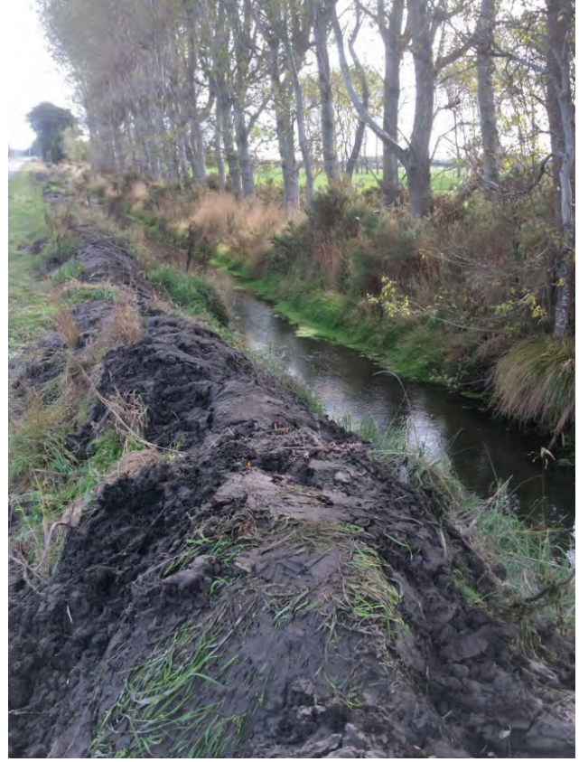
Bed (and bank material) substrate removed during drain clearing
