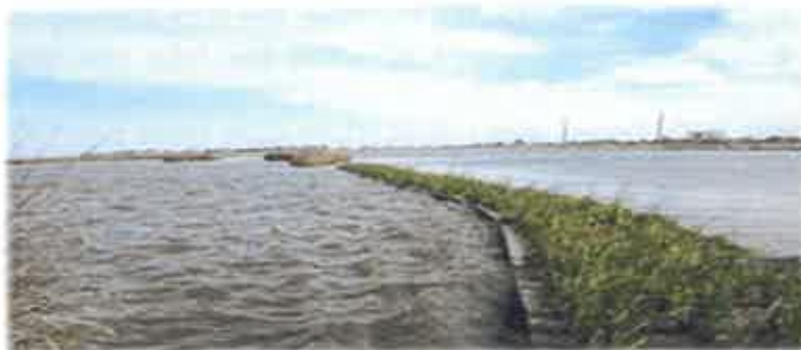
Fig 17: Floating Wetland Acting as a Wave Barrier
